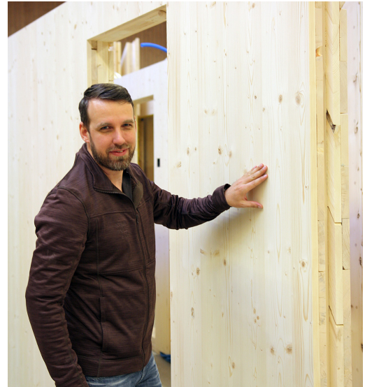
The glue-free 'Holzpur' wall elements are made from cross-laminated boards with processed surfaces.
