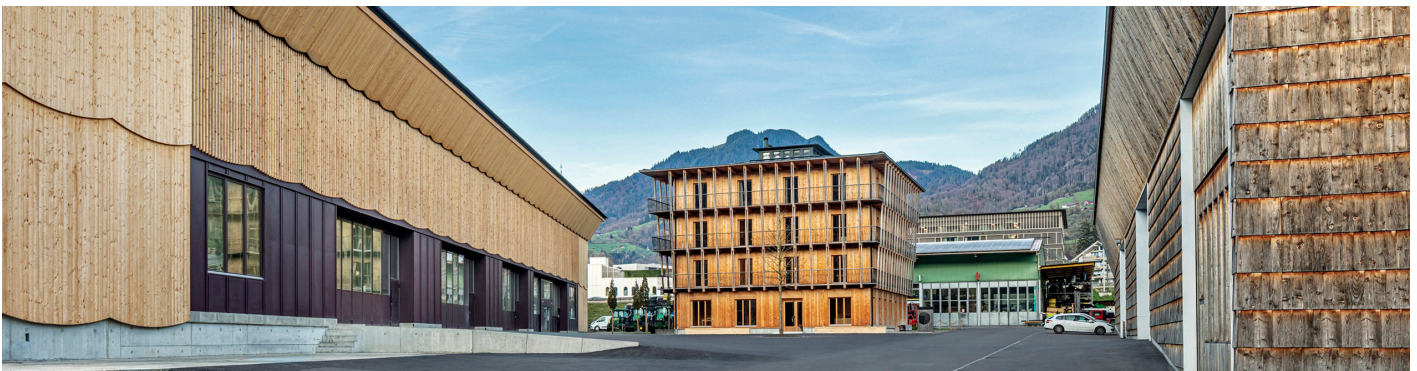
Passionate about wood construction: KÜNG HOLZBAU in Alpnach
