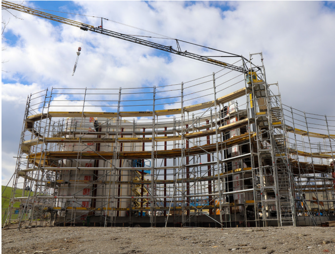
Construction progress in the past months
