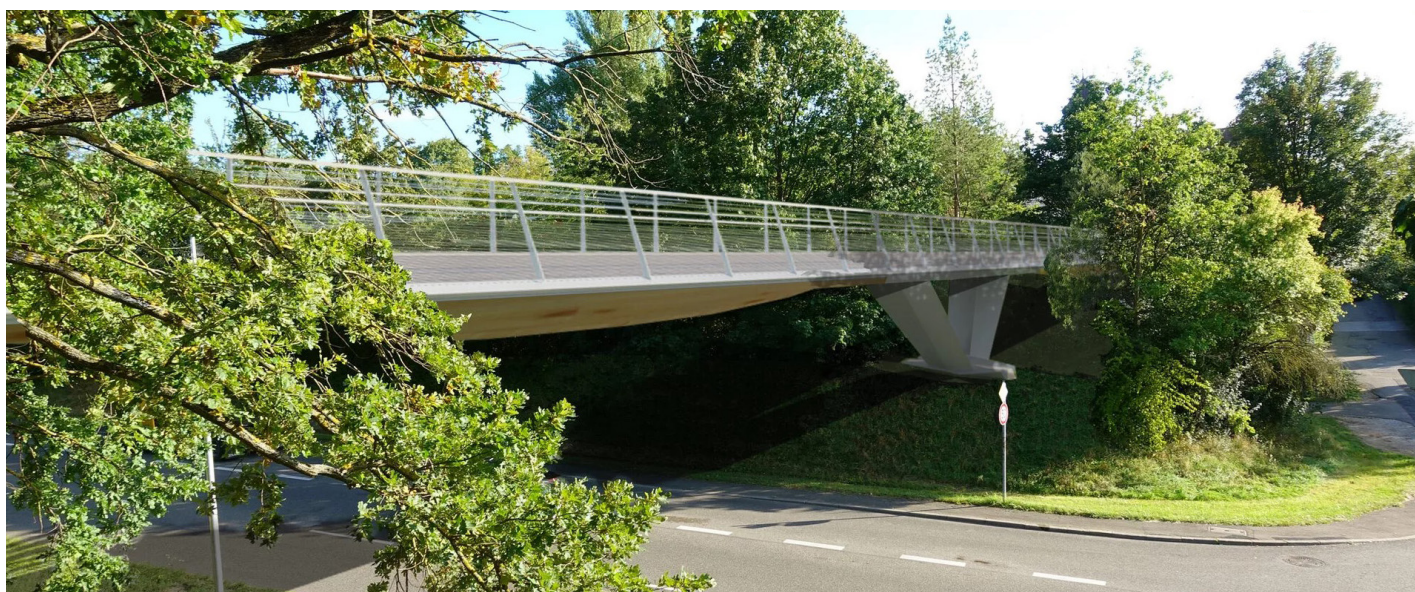
The foot and bicycle bridge has two large free form components made of glued laminated timber, which were processed on the "TW-Concept-Line" that was newly installed at Balteschwiler AG in September. Photos: Harrer Ingenieure GmbH
